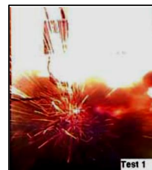
Figure 2. During test. Heater element were vaporized and contacts solidly welded. Type 1 performance.
