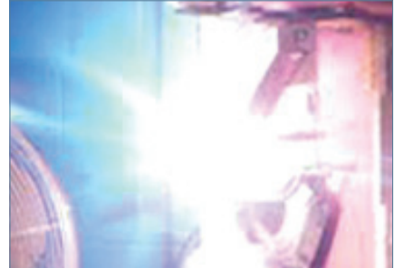
Figure 4: Case rupture of MOV during abnormal overvoltage test.
